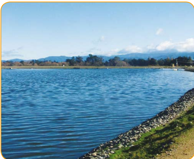
Existing treatment ponds at the Masterton plant
