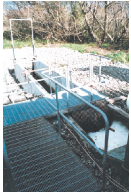
The flowmeter at the outlet to the Makoura Stream has been upgraded to improve the accuracy of monitoring.
