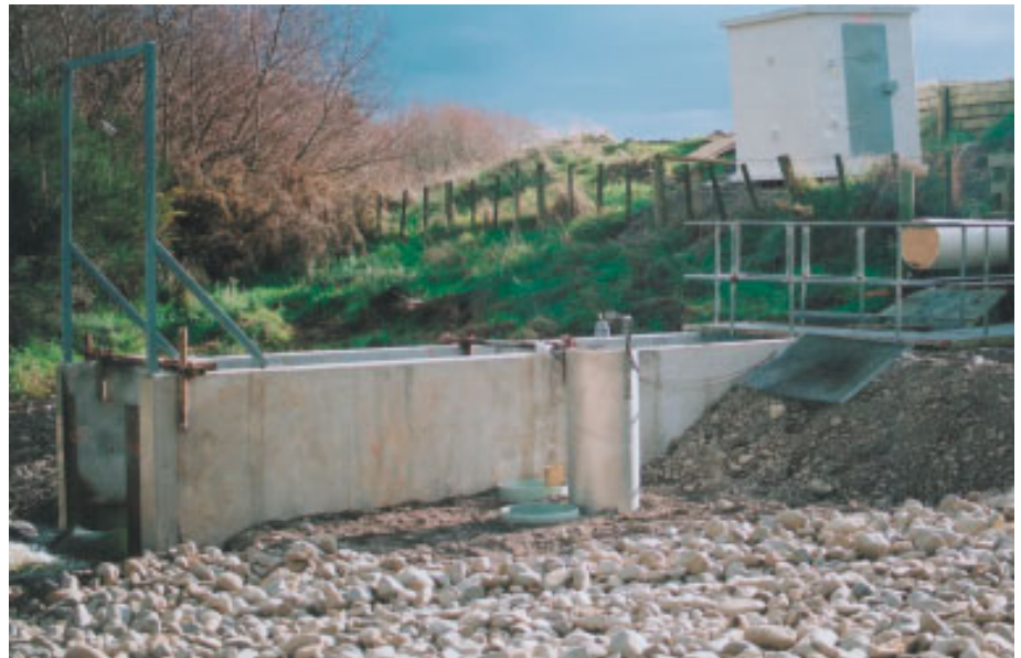
Outflow from the secondary treatment pond. The small building above houses the upgraded monitoring equipment.
