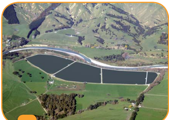
3 Existing Masterton Wastewater Treatment Ponds
