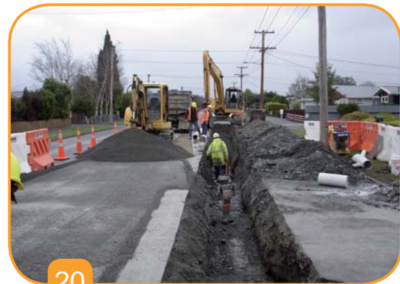
20 Cockburn Street sewer replacement
