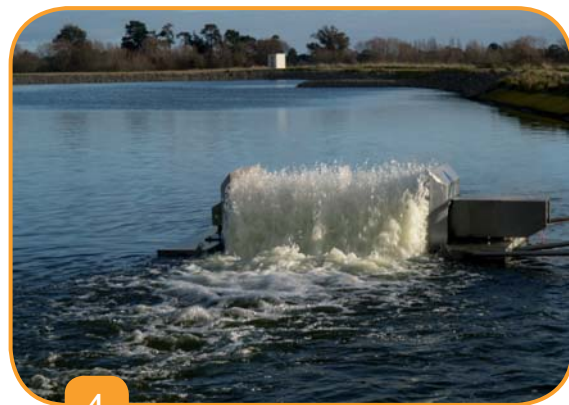
4 Aerator in the Existing Masterton Ponds
