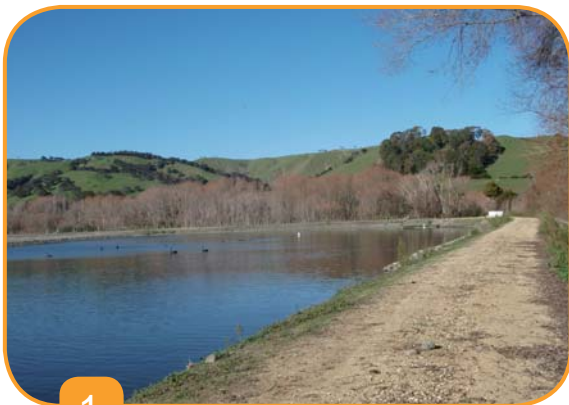
1 Existing Masterton Wastewater Treatment Ponds
