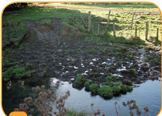
15 Existing section of the Makoura Stream with low ecological values to be diverted
